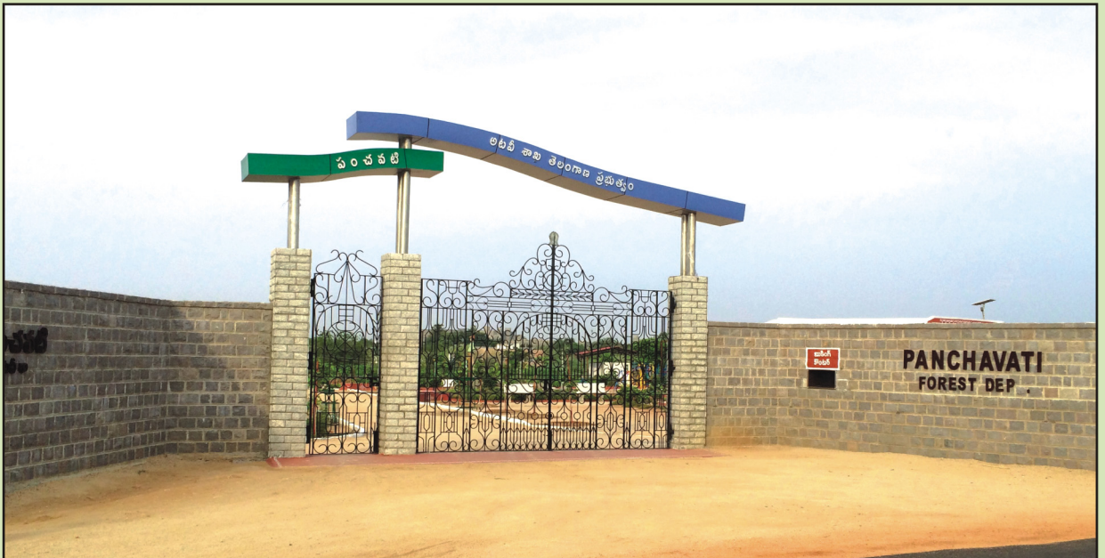
Main Entrance Gate
